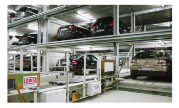
up by the transfer vehicle. After that, the Lödige Shifter will take you to a free parking space. And at the end of the parking period, the car is automatically transported back up at the push of a button.
