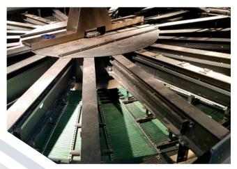
The slip rings are divided into segments and provide the complete power supply for the huge revolving stage. They transmit electric power for everything that is needed on stage: from filming and scenery to lighting, video, and sound. Likewise, rectangular elements can be raised and lowered on the stage. The VAHLE slip rings were installed in the fall of 2005 and have only been dismantled and reinstalled once. They have been in operation ever since without any modification or maintenance.
